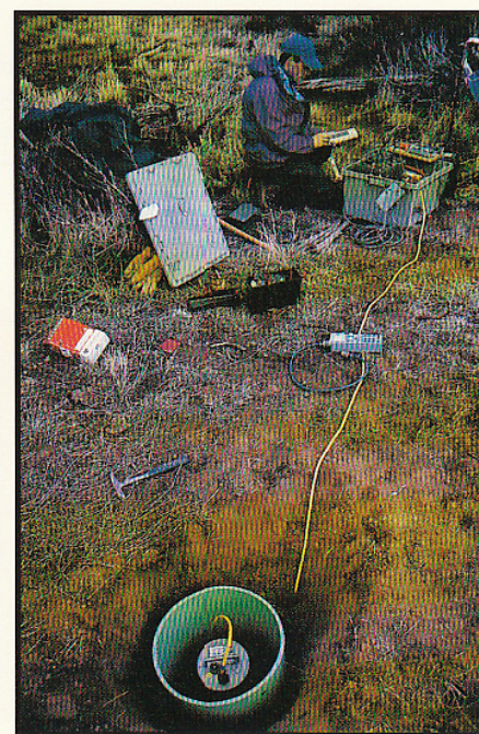
Figure 2b. Installing station CYF. Typical CPGB installation using sewer pipe for vault is apparent. Colcrado University-Boulder undergraduate Ncah Hughes is examining the recording equipment.
